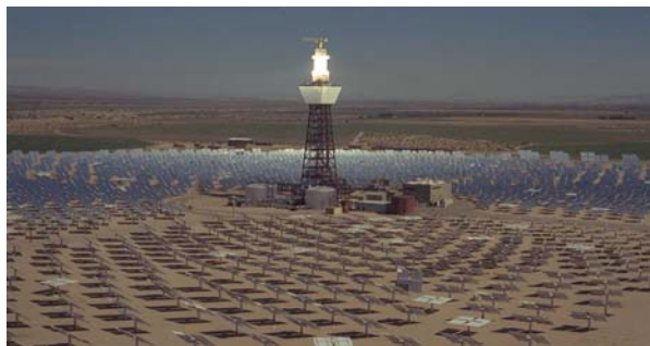
Solar Power Tower
