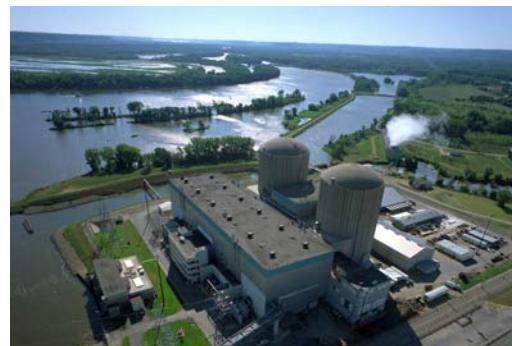
Thermoelectric Power Plant
